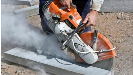
Figure 1 Dust cloud created by cutting concrete
